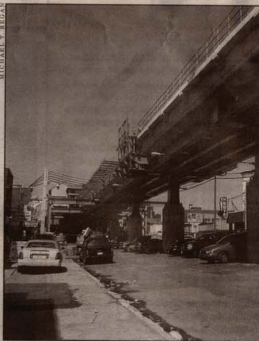
THE BIG PIG: Originally estimated at $420 million, SEPTA's EI project has nearly doubled in cost.
